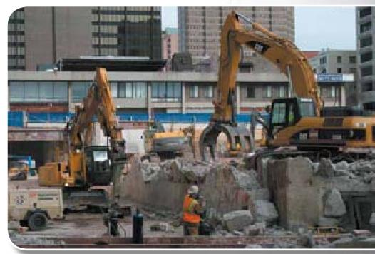
Worker wearing respirator observes demolition of New Haven truck tunnel by Laydon Industries' CAT 330D, John Deere 210C and Volvo EC360B excavators.
