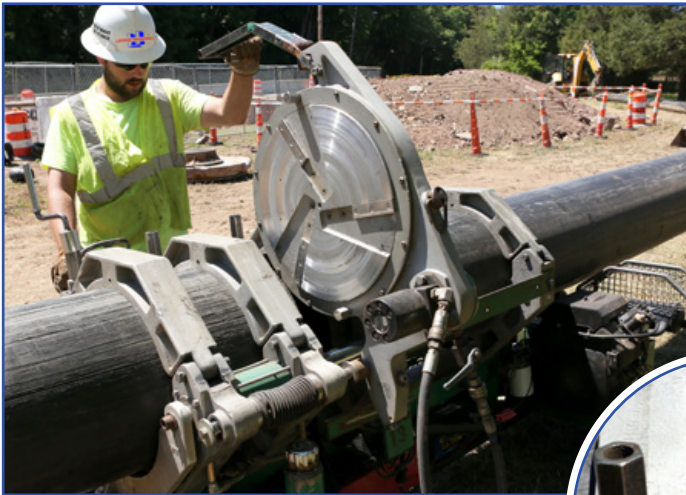
Plastic line piping sections are cut and then welded via a high heat fusion process.
