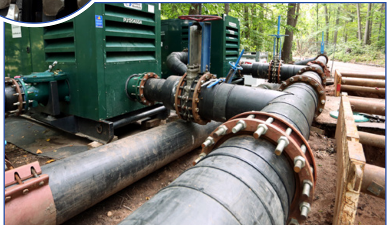
Straight and radius piping configurations are custom fabricated onsite.
