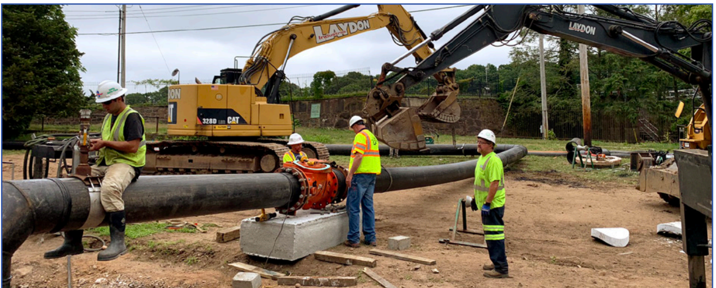
Crews working on assembling the semi-permanent 18" HDPE bypass line.
